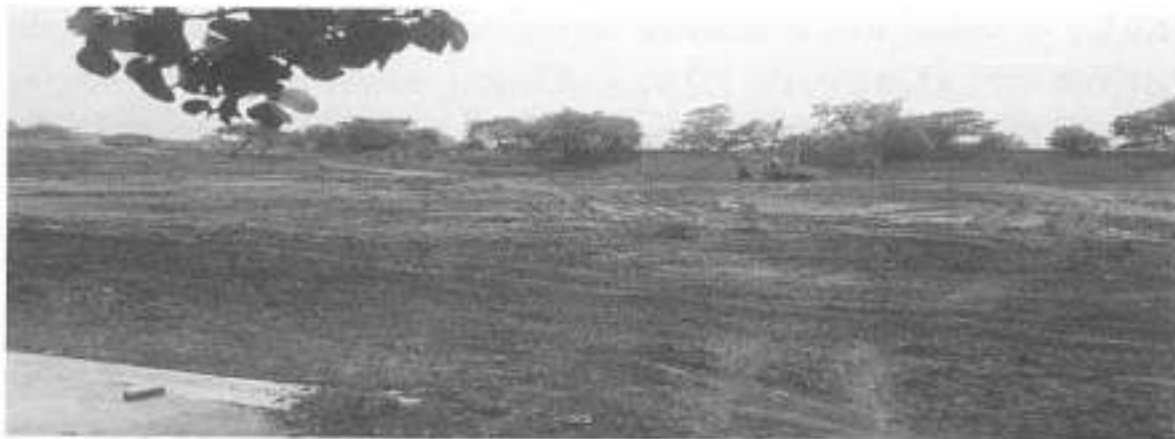
Photo 12: Cleaning and deepening work of Dadu Pond at Village Badadarha has been completed to enhance water storage capacity and improve overall water resource management
