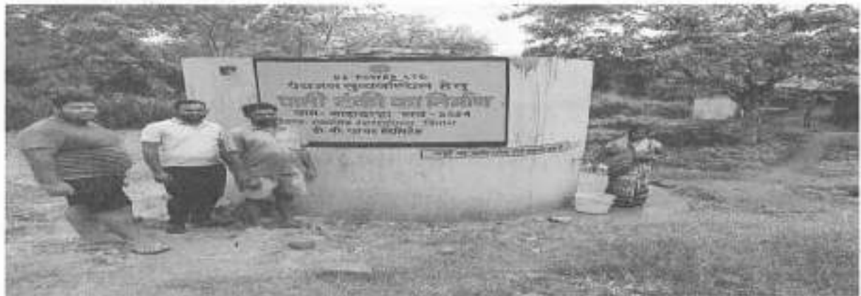
Photo 3: Construction of a 10,000-litre capacity water tank at Beech Basti, Village Badadarha, to strengthen local water infrastructure.
