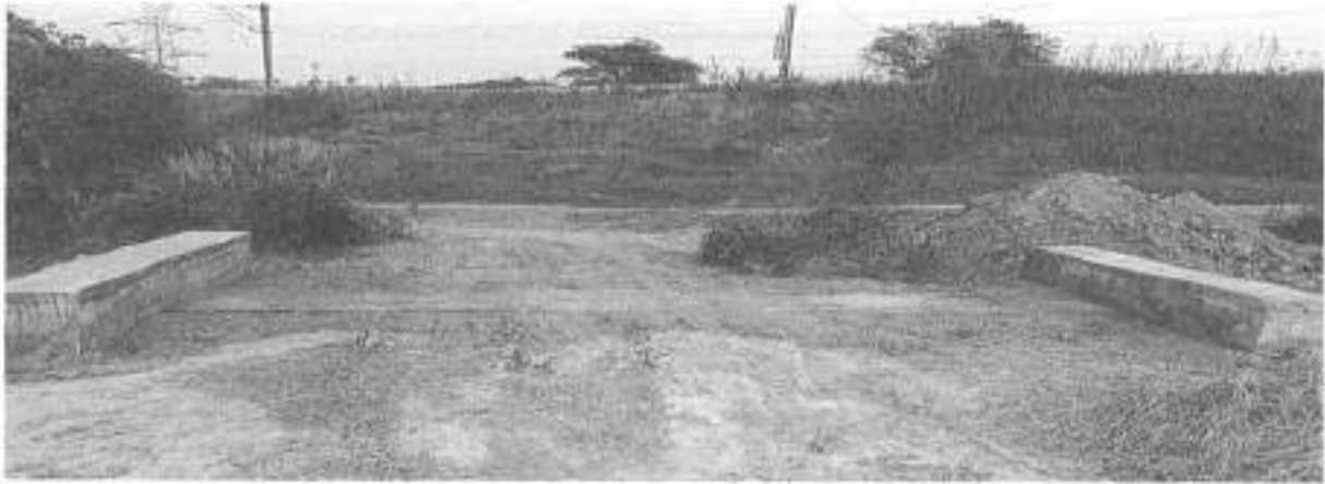
Photo 10: A Hume pipe culvert has been constructed on the bypass road connecting Fulbandhiya to Khairpali.
