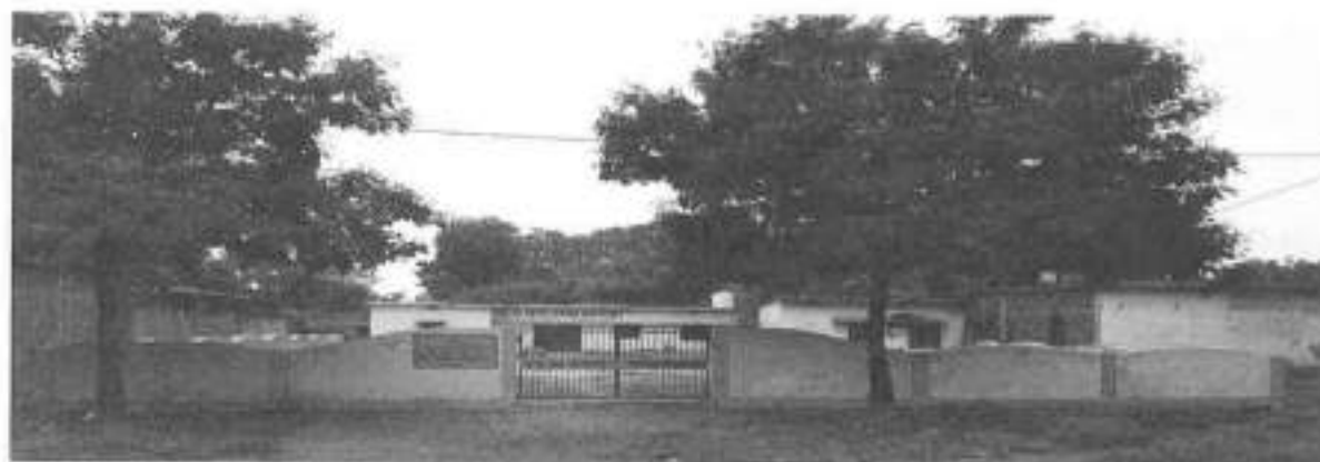
Photo 5: The boundary wall of the Government Primary School at Rampur and the backside boundary wall of the Government Higher Secondary School at Tundla
