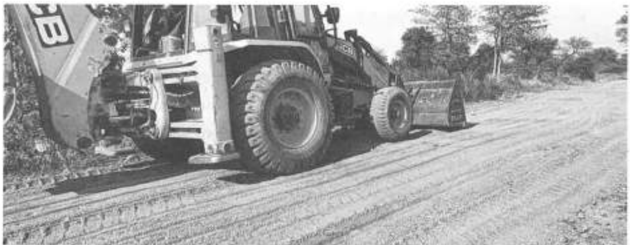
Photo 11: The bypass road connecting Fulbandhiya to Khairpali has been repaired and strengthened with murum to improve connectivity and ensure smoother transportation
