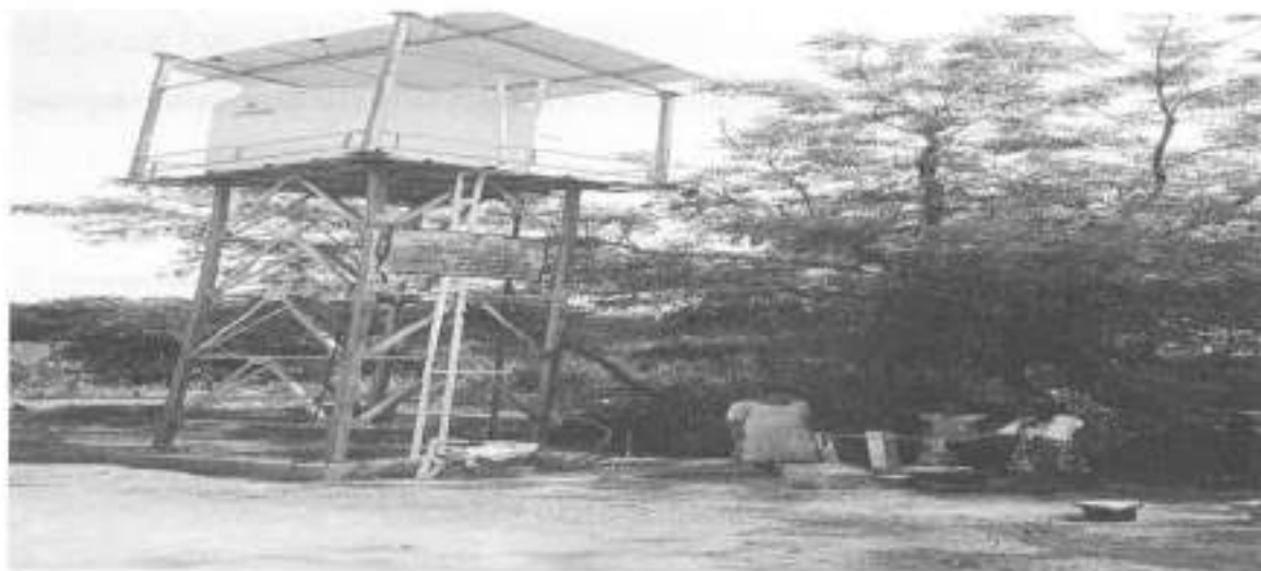
Photo 2: The Solar-Powered Drinking Water System has been installed at Rampur, Badadarha.
