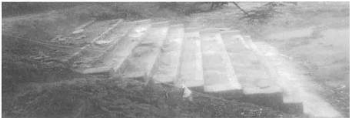
Photo 8: Existing bathing steps at Dadu Pond in Village Badadarha have been repaired to improve safety and accessibility for the community.
