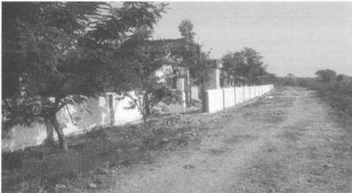
Photo 6: The boundary wall of the Government Primary School at Amapali has been constructed to ensure a secure and well-defined school
