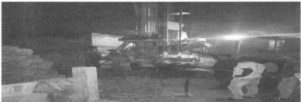
Photo 4: Borewell drilling completed at Mahant Mohalla, Badadarha, ensuring reliable water supply for the community.
