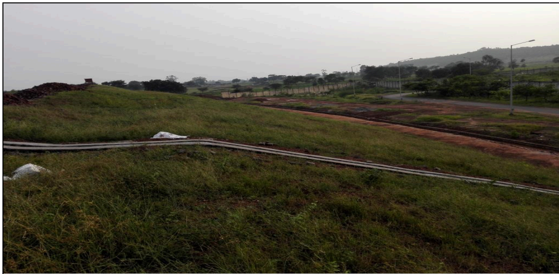
Figure 22(e) Slope drain. Size - Wide 300mm & Depth 200mm
