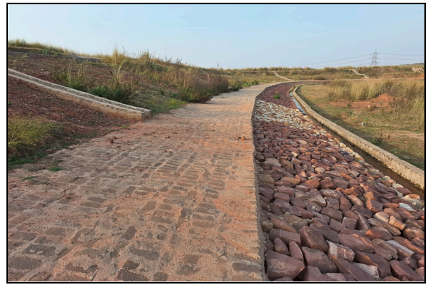
Figure 27(f) Rock Toe filter.
