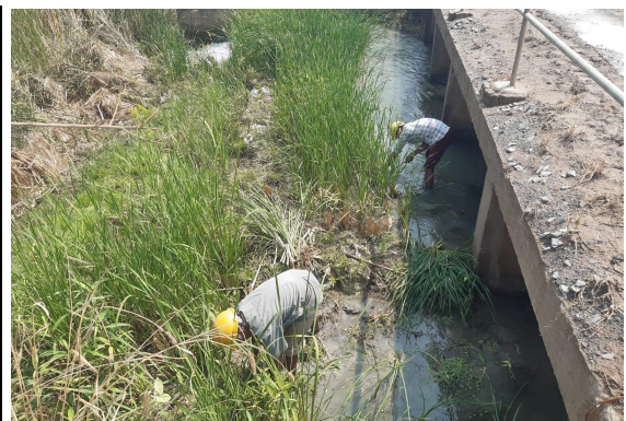
Figure 27(h): Cleaning of the spillway
