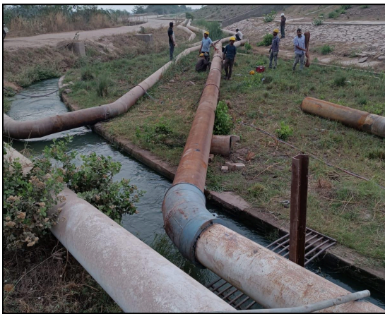
Figure 27(c) Ash slurry pipes after repairing work.
