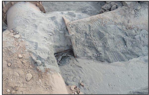
Figure 27(C) Ash slurry pipes before repairing work.
