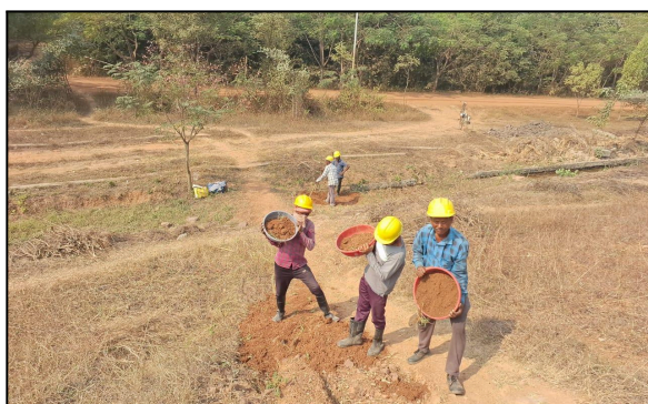
Figure 23: Rain cuts filling work
