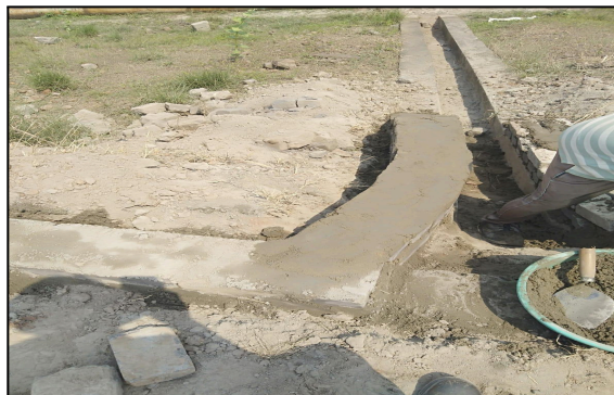
Figure 24: Slope drain repairing work
