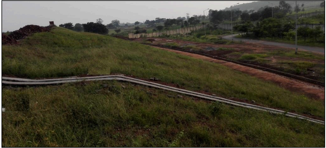
Figure 18: Slope Drain and D/S side slop Cover with Turfing. Rectangular strips of uniform width, not less than about 25 cm x 30 cm in size.
