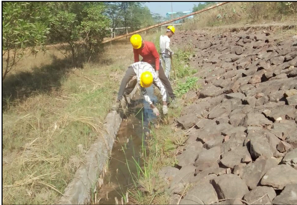
Figure 27(e) Cleaning of Toe drain.
