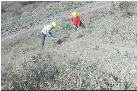
Figure 27(b) Vegetation clearance
