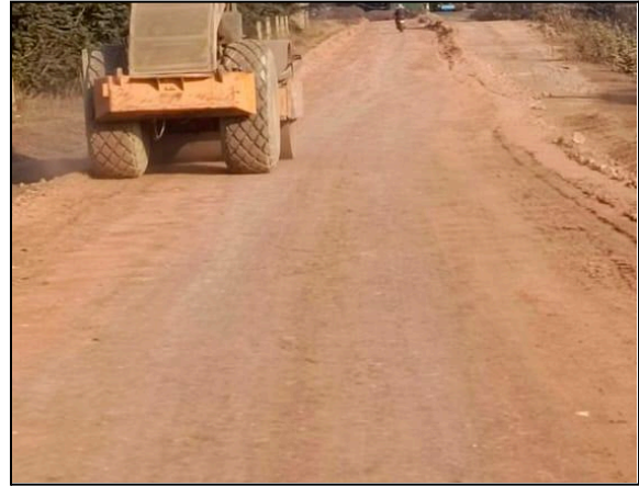
Figure 27(a) Road repairing work (other action)
