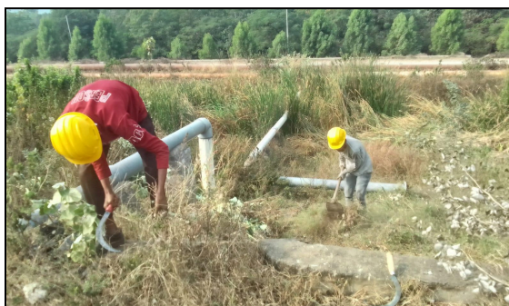
Figure 26: Vegetation cleaning work
